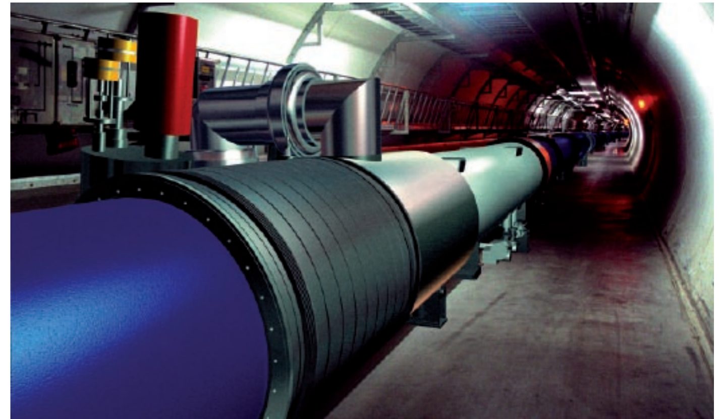
The LHC tunnel
